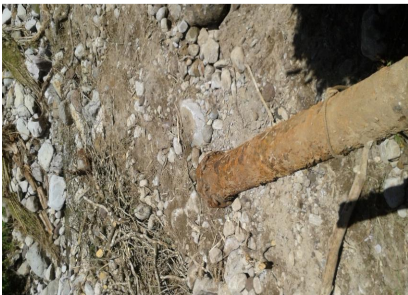
Broken pipeline at Pichelin
