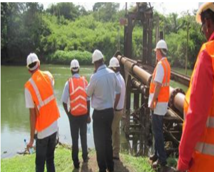
Team Inspecting Surface Water Intake at the Belize River
