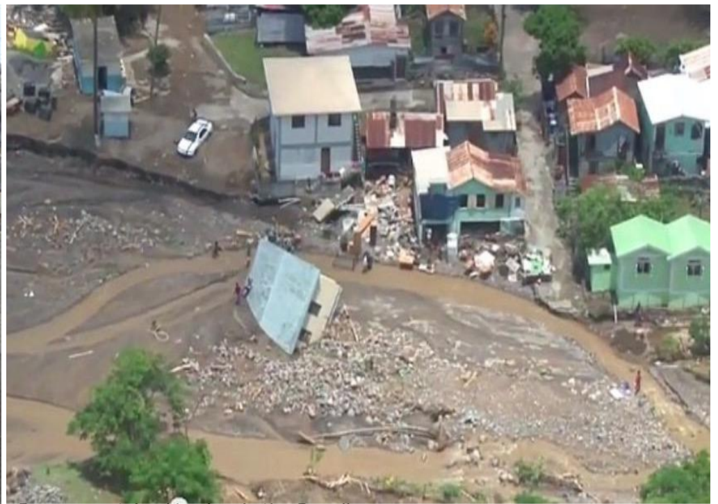
Damage sustained by river in the Grandbay area
