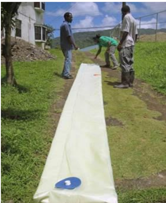
Inflatable plastic bag digester
