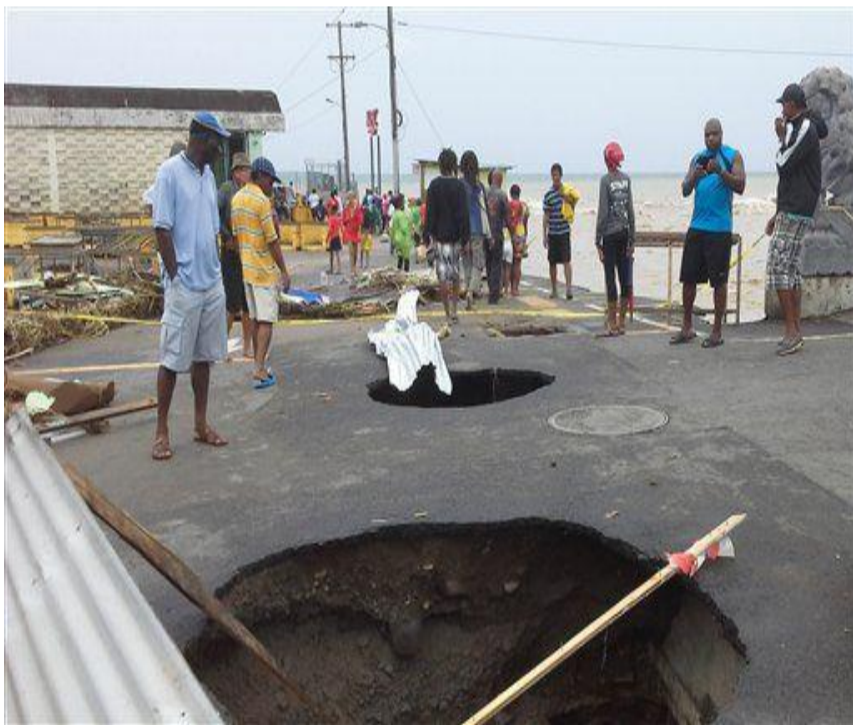
Sewer Collapse on the Roseau Collection system
