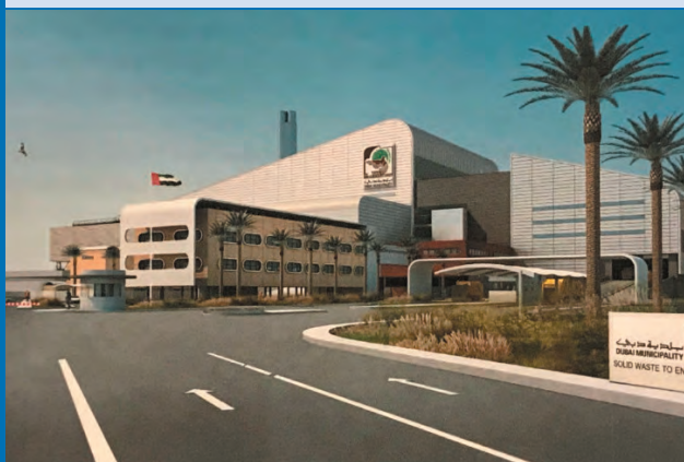
Dubai WtE plant.
