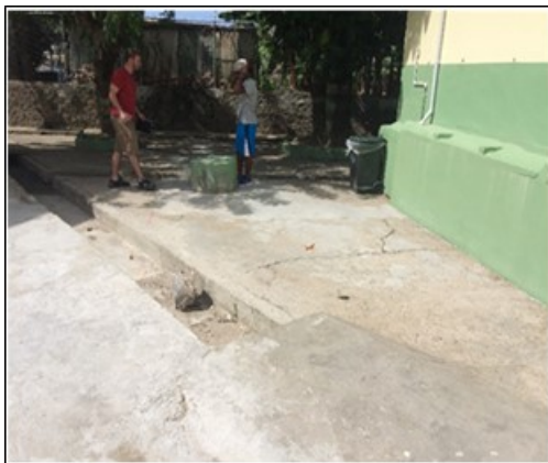
The primary school had a new septic tank installed within the last 2 years. It has not been pumped to date. It appears to discharge into the open gutters.
