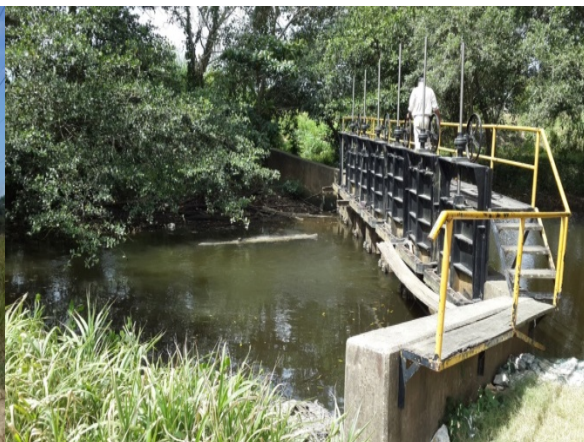
Ineffective sluice gate system used to control tidal flow
