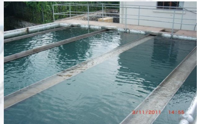
Settling tank old plant with new weirs
