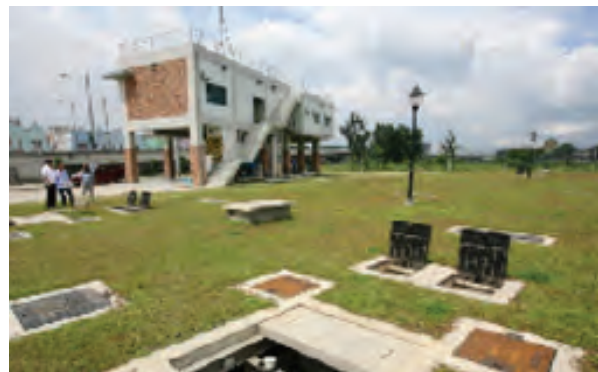
Olandes STP (Marikina City): process tanks built underground and support facility on stilts (Source: Steve Griffiths)
