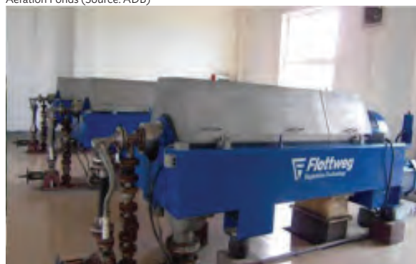
Sludge-Dewatering Centrifuges (Source: ADB)
