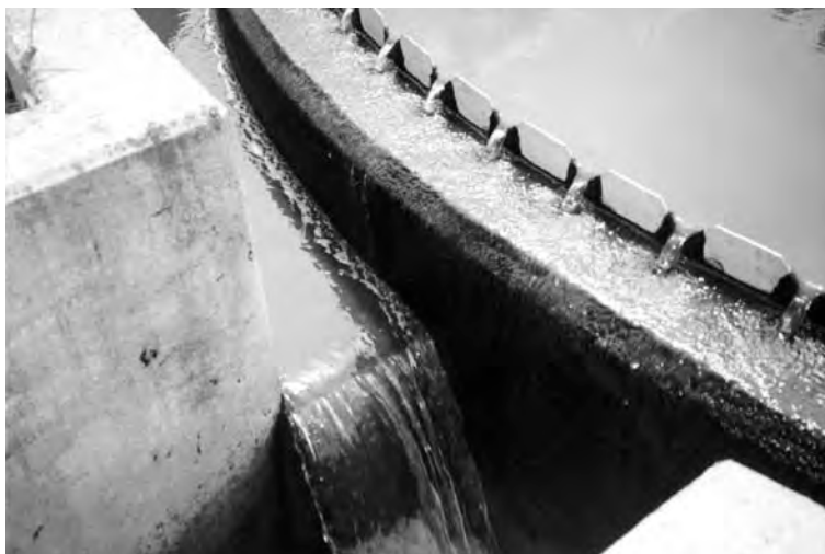
Effluent from the secondary sedimentation tanks at the Arima sewage treatment works.
