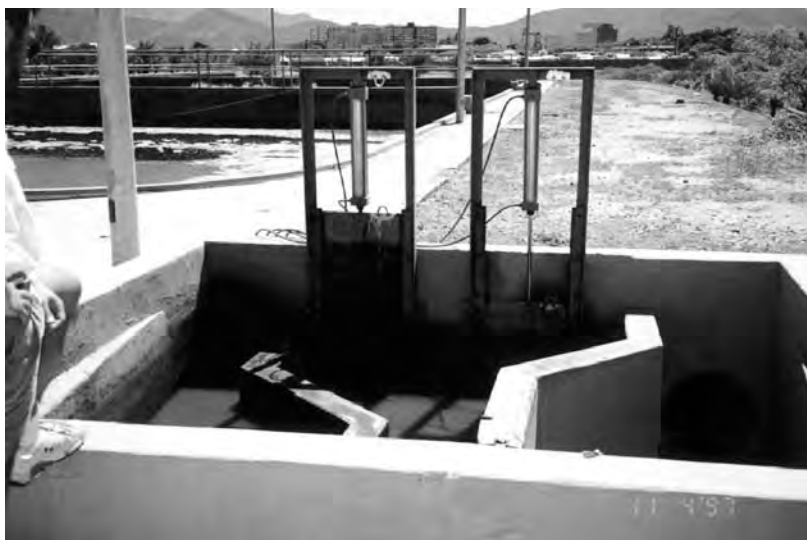
Simple pneumatically operated gates cyclically feed different zones of the MSBR at the Juangriego treatment plant.
