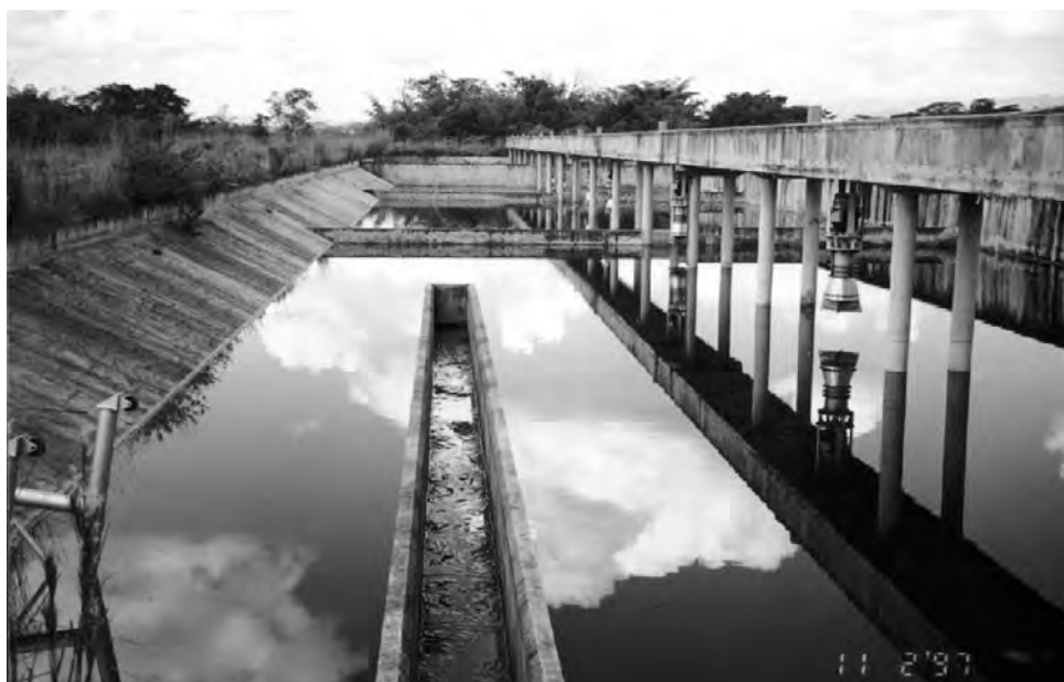
MSBR tanks at the Mariposa treatment plant will use high-speed direct-drive propeller aerators suspended from concrete access bridges.
