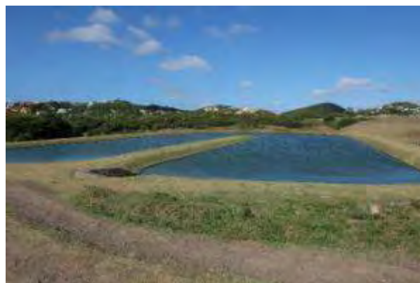
Picture 18: Facultative Aerobic Pond at Beausejour WWTP
