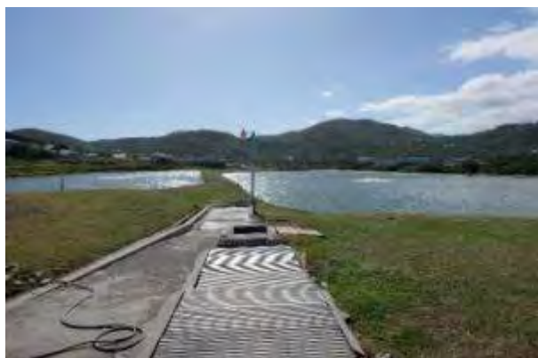
Picture 19: Aerated Ponds at Beausejour WWTP
