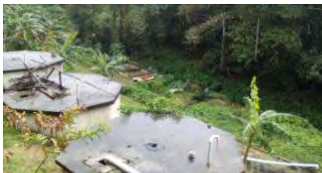
Picture 16: CCC FSTP at Union
