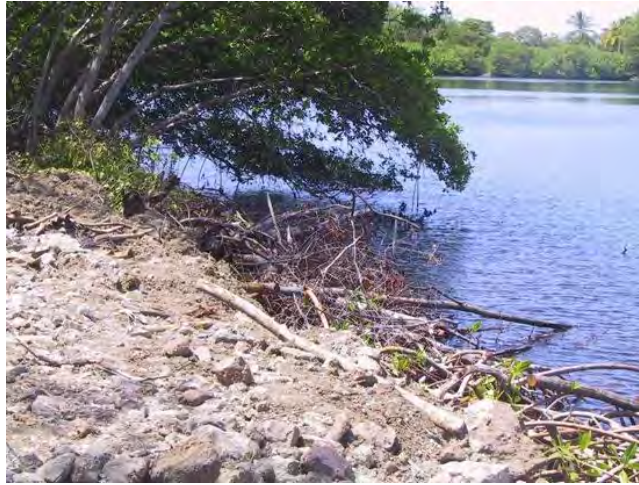
Figure 4.2: Encroachment into mangrove forest
