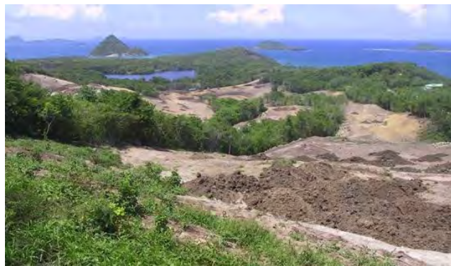
Figure 4.4: Littoral forest being cleared for development, Levera
