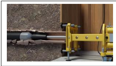
Figure 9 Pipe Bursting Head & Hydraulic Thruster
