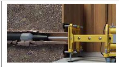
Figure 9 Pipe Bursting Head & Hydraulic Thruster
