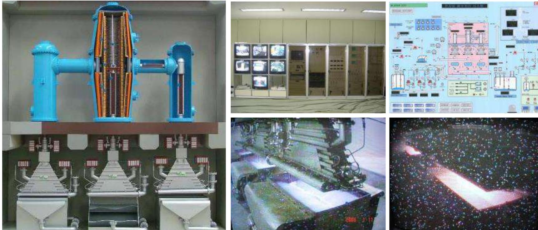
Full-scale application of electron beam wastewater treatment plant for 10,000 m<sup>3</sup>/d of textile dyeing wastewater with 1 MeV, 400 kW accelerator.
