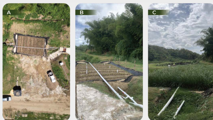
Figure 1. A) Drone shot of Constructed Wetland, note overflow pipe passing on surface of wetland. B) CW after installation of vetiver plants on 19th January 2024. Note 6 vertical perforated pipes for air flow/access into the substrate. C) CW on 5th June 2024, note the growth of vetiver grass.
