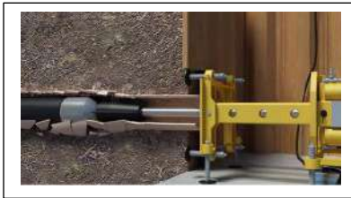
Figure 9 Pipe Bursting Head & Hydraulic Thruster
