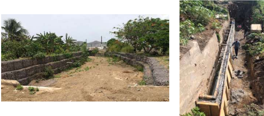
Figure 2. Gabion baskets installed (left) and weir repair (right)
