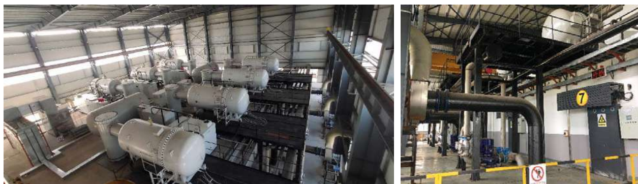
FIG. 3. Treatment plant in China uses electron beam to treat wastewater from textile industries.
