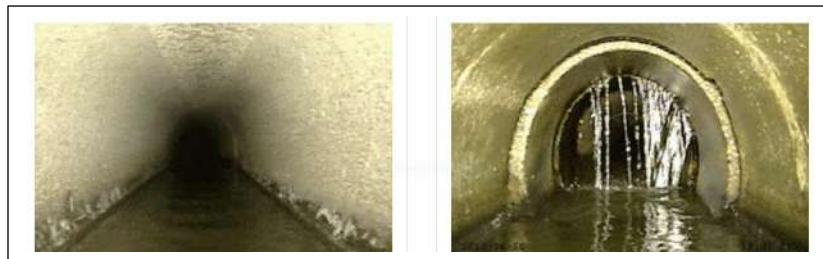
Figure 2 Inflow & Infiltration in a 18inch Waste water pipe
