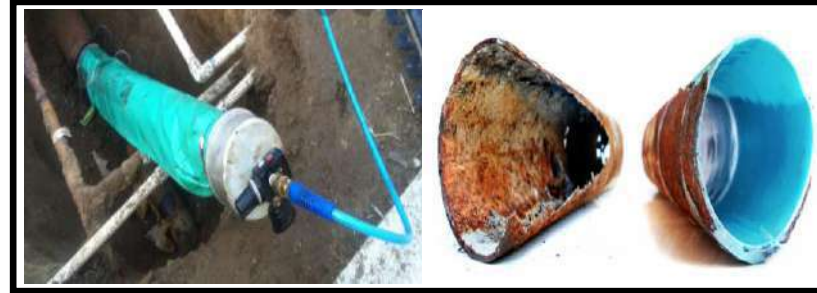
FIPP Pipe Liner 1992/1993
