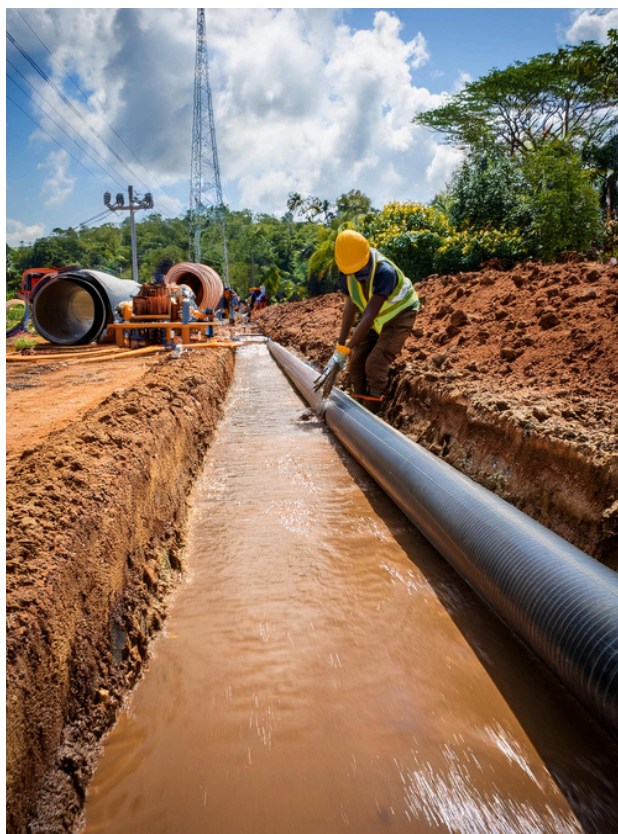
Laying of pipes. Adobe Firefly
